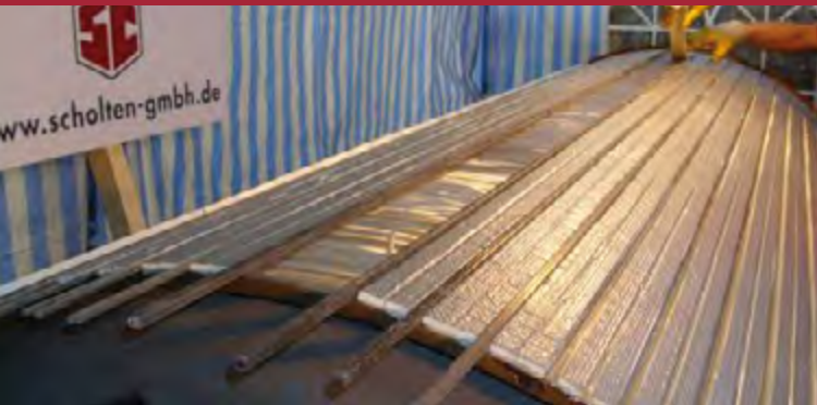
Special bonding procedure in a construction tent
