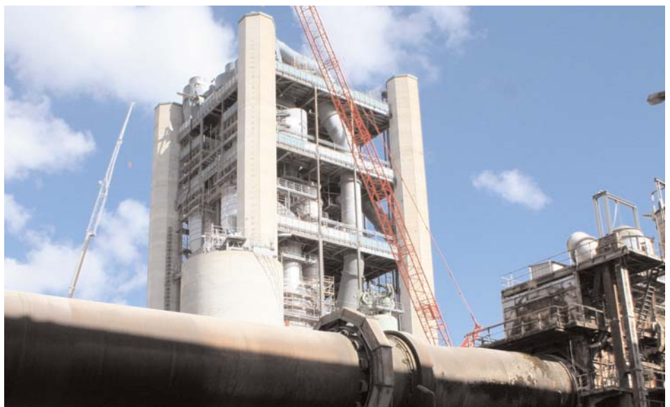
The riser dryer in the Lägerdorf plant has a height of 60 metres.
