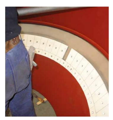
The term ,alumina ceramic' defines ceramic materials with an aluminium oxide  $(Al_2O_3)$  content above 80 %. (Generally, only ceramics with a minimum  $Al_2O_3$  content of 92 % should be used as high-quality wear protection.)
