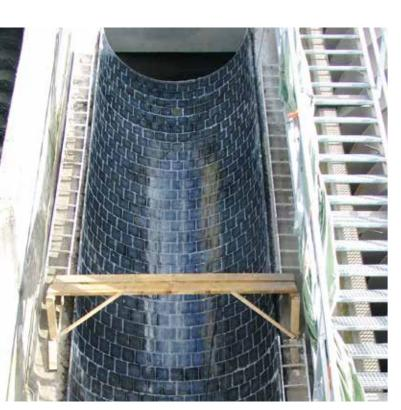
Cast basalt is a mineral material which, thanks to its special characteristics, is superbly suitable as wear protection:
