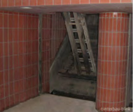
Floor and side wall linings with cast basalt (pictured left) or with hard ceramic (pictured above).
